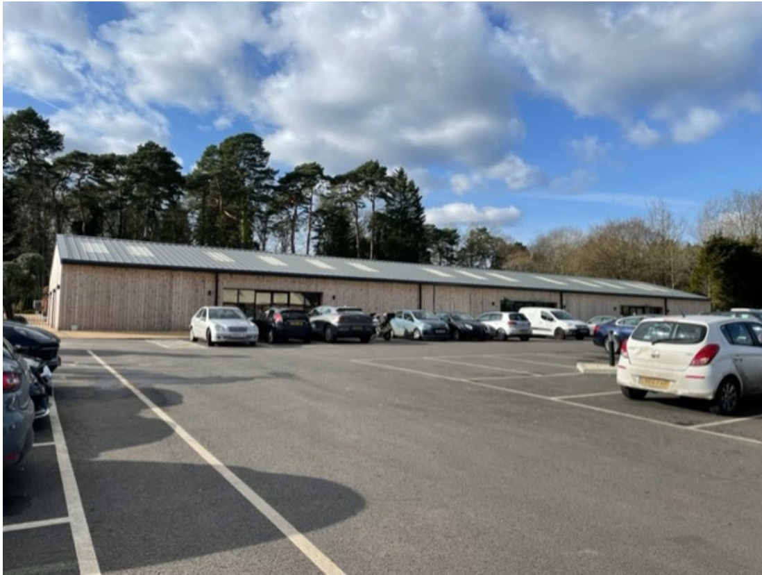
Front elevation and car park
